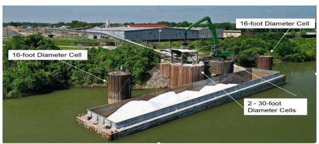
There are three barge cells that are only accessible by water. The cells can be accessed via exterior ladders to gain access to the top of the cells. Two cells are located at the GCB and one cell is located at the BCB. They are identified in the following picture.
